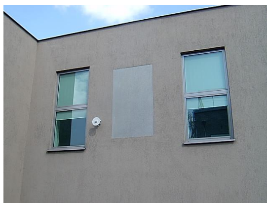
Figure 1. South oriented wall of the tested space with two windows and the transparent insulation panel in between
